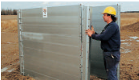
Corner end-posts are pinned in place.
